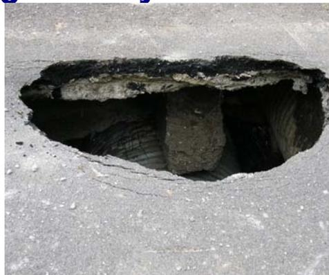
The county-maintained bridge on Naylor road, just south of Cross Roads town limits, was left impassable following rains that washed out the substructure. A huge crevasse remains where rock used to be compacted over culverts. For further information, contact the county commissioner for Precinct 1, Cynthia White, at 940-349-2810.
